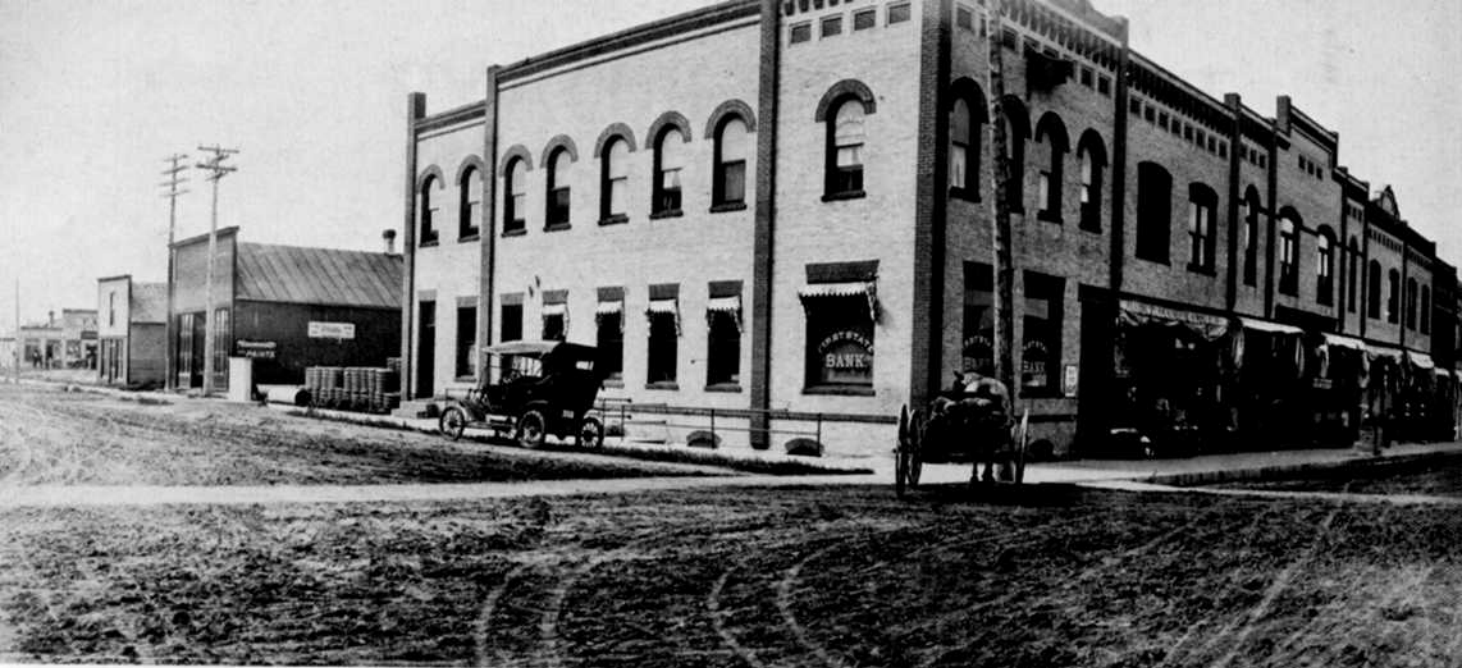
Main Avenue looking north from Second Street about 1912. Brick Block built in 1897 is to the left, the Kaus Block on the right.
