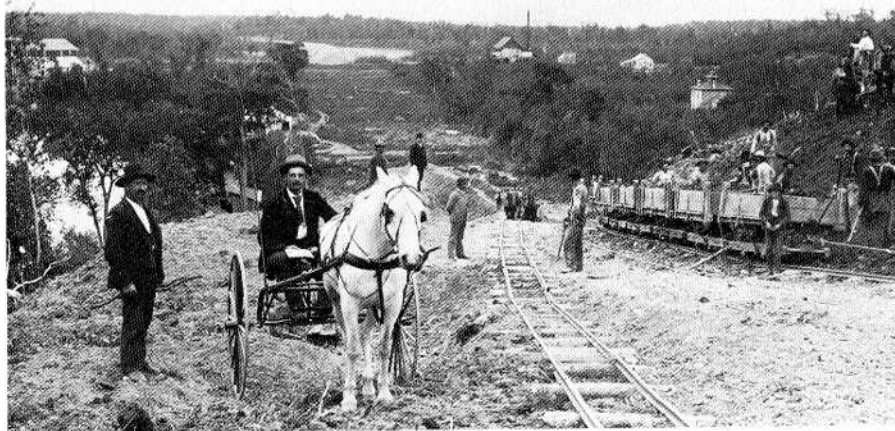
Building the road bed to the Red Lake Falls Milling Company.
